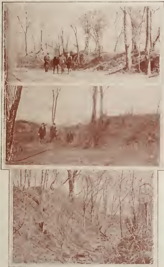
PRESENT CONDITIONS ON FORT FIGURES.
